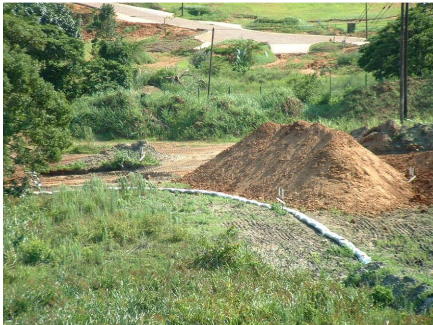
Sandbag berms and cladding has prevented slumping of soils into conservation area.
